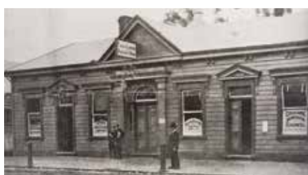
First library, Lowe Street, Gisborne
