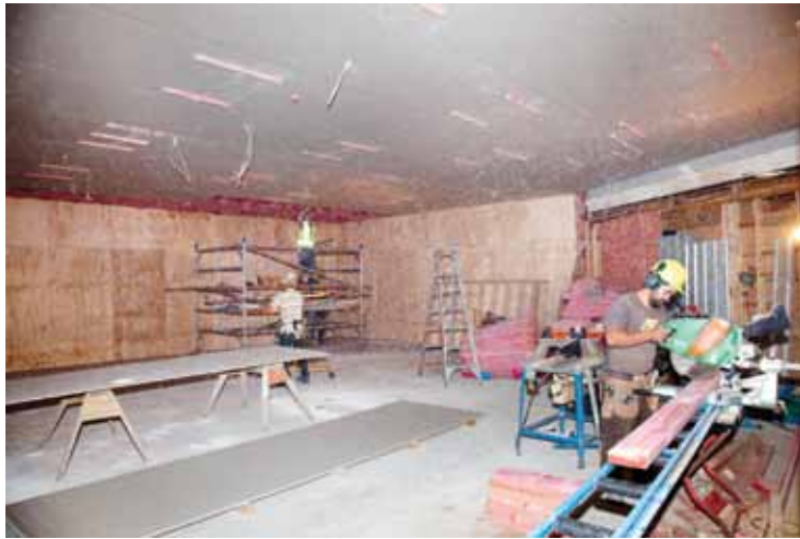
Museum extension construction
