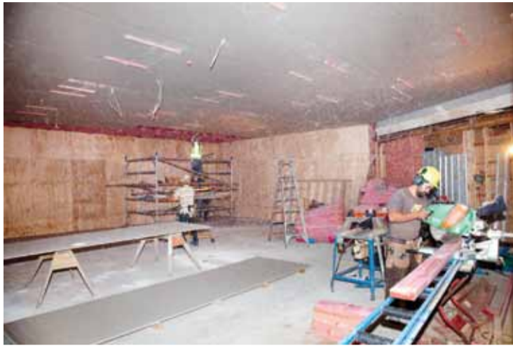
Museum extension construction
